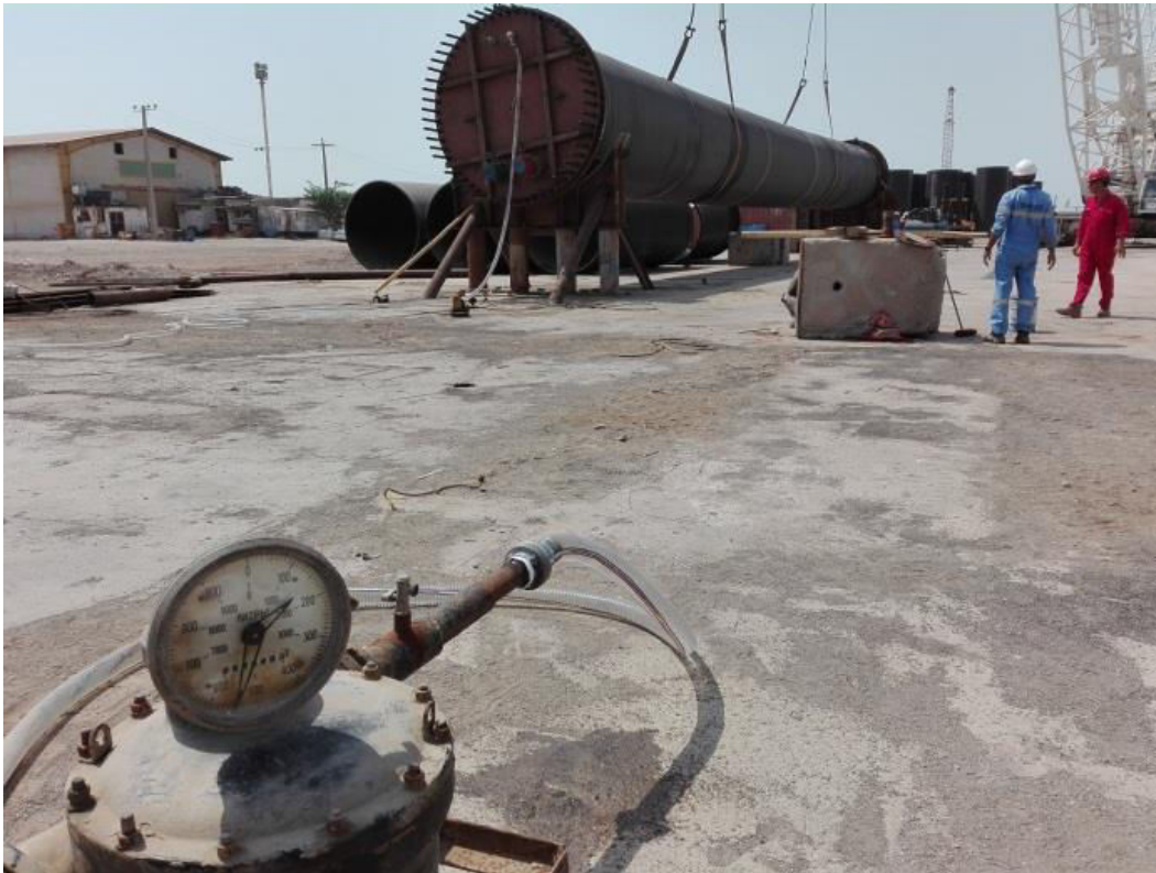
Figure 11. Injection water hose and flow meter view
