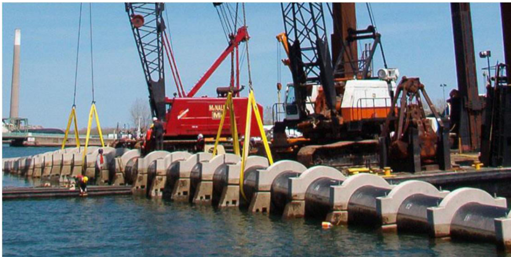
Figure 2. Typical view of the Installed Concrete Ballasts
